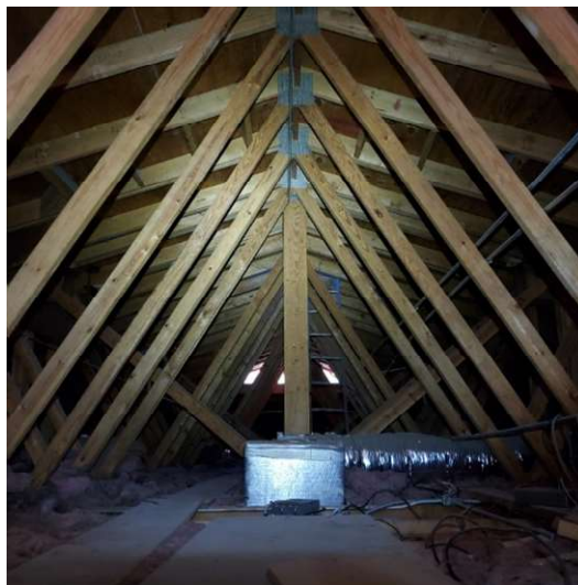
Figure 34: Attic Space – Wood Truss
