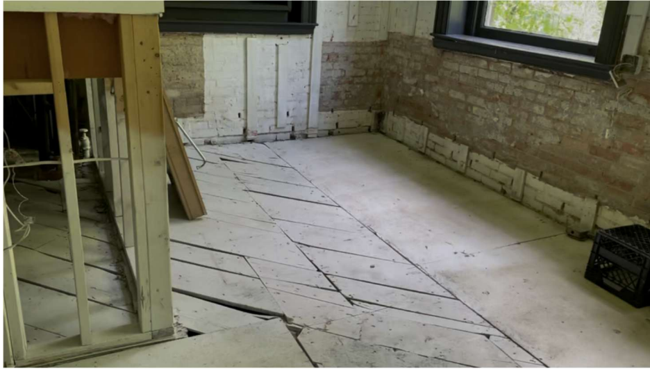
Figure 26: First Floor - Rear Room – Mix of Plank Floorboards and Sheathing
