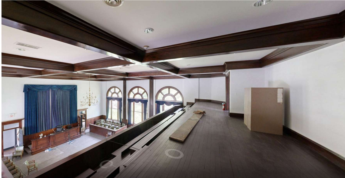
Figure 10: Existing interior balcony level.
